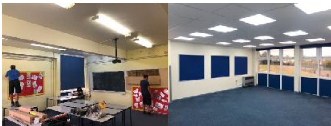
Classroom before lights and acoustic tiles
